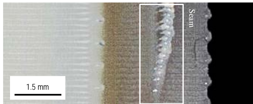
Fig. 10: Building defects on the outer wall through uncontrolled delivery of material
