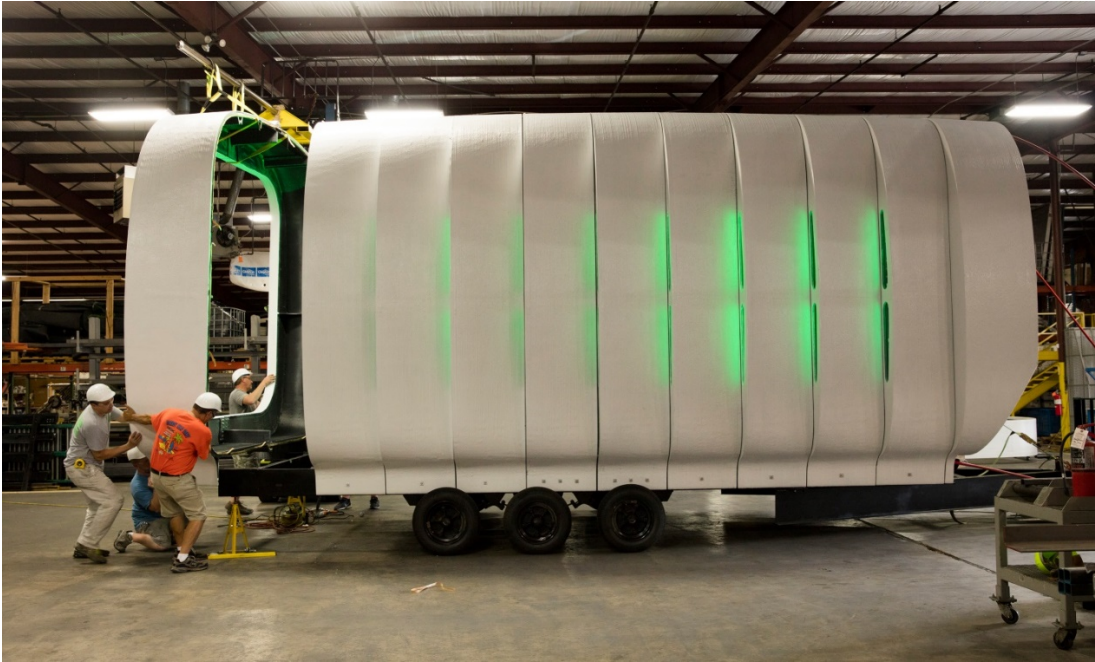
Figure 6: Sections of the Project AMIE House During Assembly.
