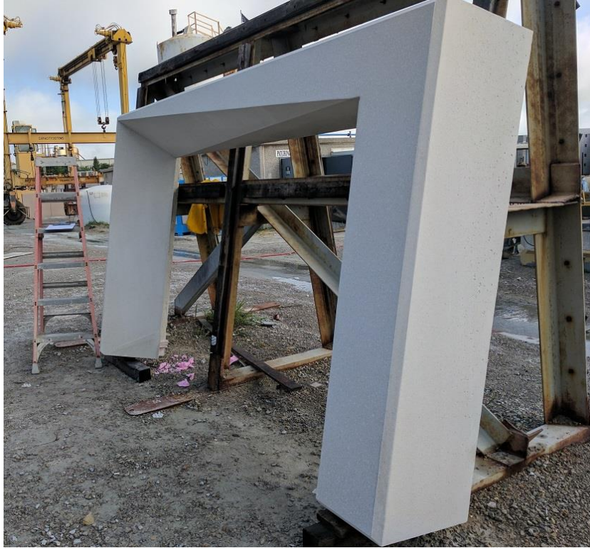
Figure 15: A completed concrete part that has been pulled from the mold
