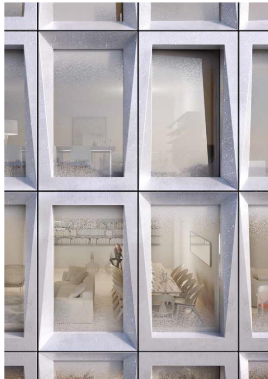
Figure 4: Rendering of the concrete patterns with inset windows
