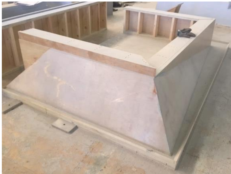
Figure 2: A traditional manufactured concrete mold using wood
