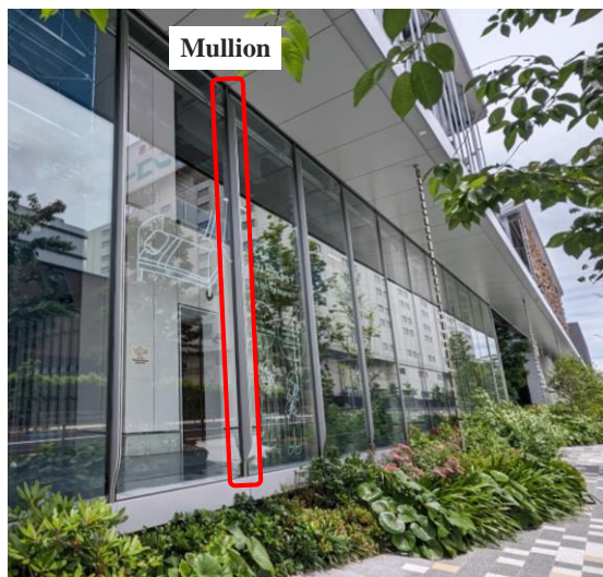
Figure 1 Aluminum mullions used in architectural facades
